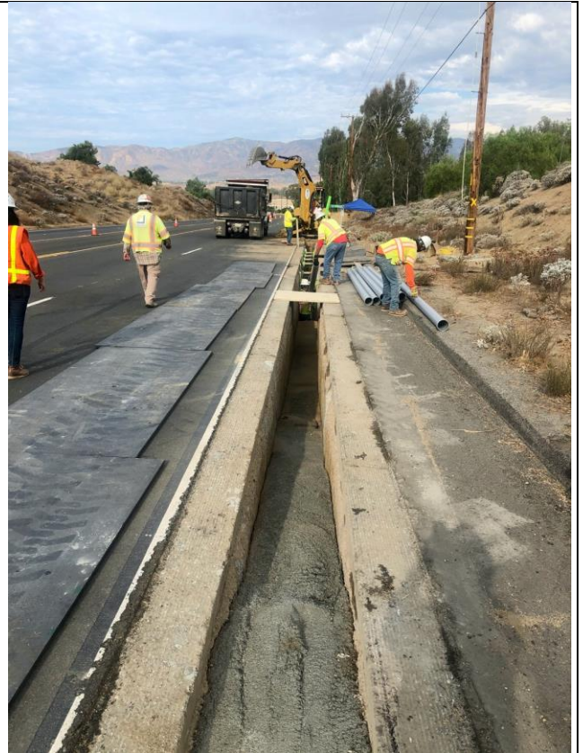
Figure 3. Conduit installation along State Route (SR) 74, August 23, 2020
