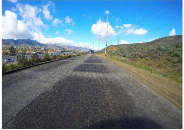
Concordia Ranch Rd. Photo taken on February 23, 2022, facing northwest.
