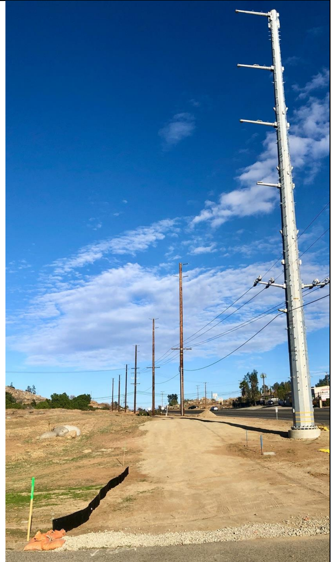
Figure 6. Newly installed TSP 45 with BMPs, January 20, 2021
