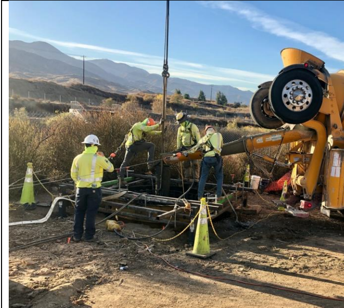
Figure 5. Concrete pour of TSP 449, December 16, 2020
