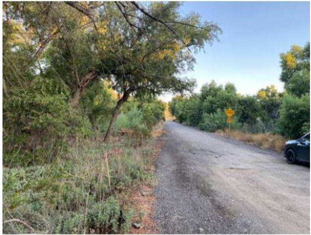
Feature ID: 41. View of work area and southern arroyo willow riparian forest prior to tree trimming. Photo taken on July 29, 2021, facing northwest.
