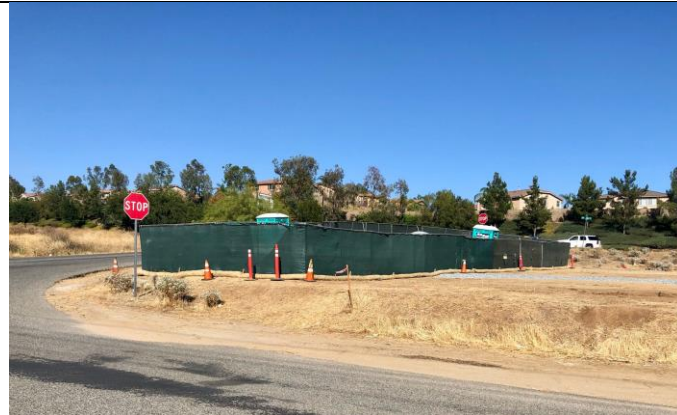
Figure 2. Perimeter fencing established at the 74 Central Yard, July 21, 2020
