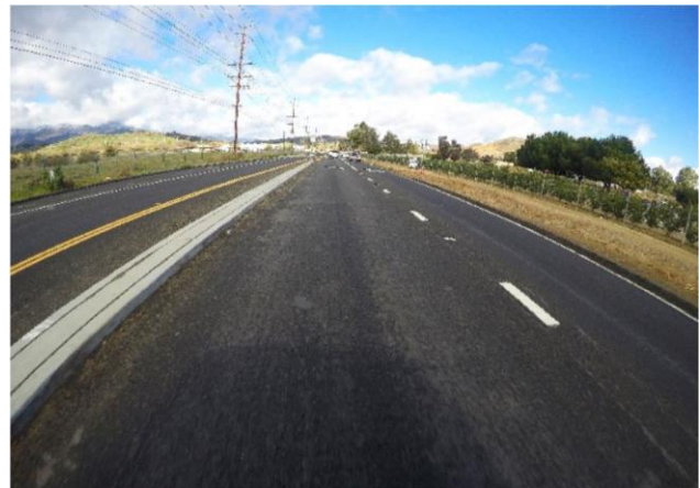
Collier Ave. Photo taken on February 23, 2022, facing northwest.
