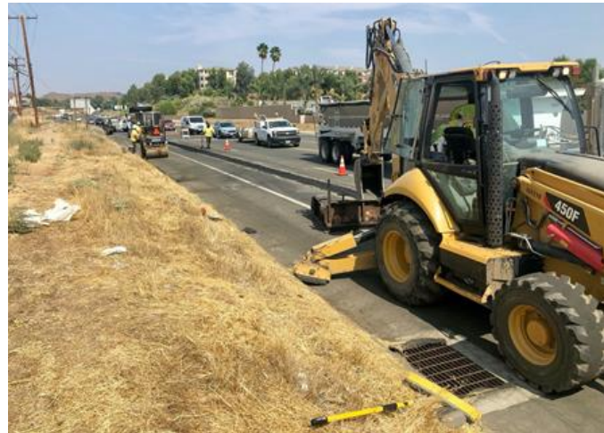
Figure 4. Paving along SR 74, September 17, 2020
