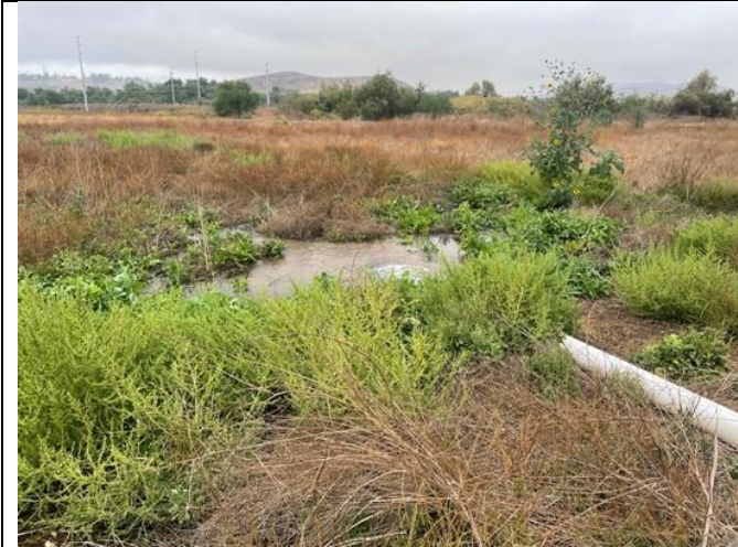
Figure 11. Discharge area for the dewatering operation in Segment VIG4, October 6, 2021
