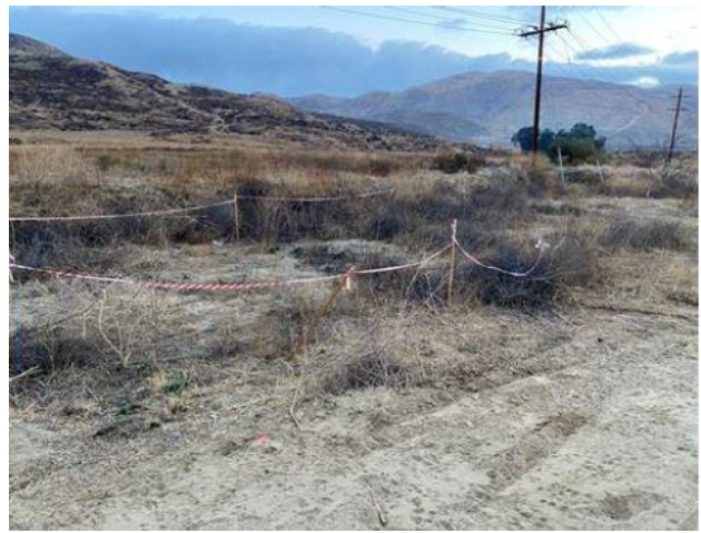
Feature ID: 50. View of work area and ephemeral drainage at Pole 4765413E pre-construction. Photo taken on December 3, 2021, facing northeast.
