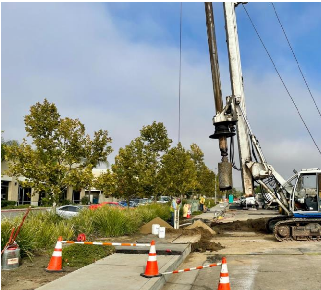
Figure 10. Drilling at Pasadena St. prior to vault installation, September 16, 2021
