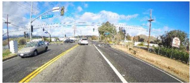
Intersection at Collier Ave. and Riverside Dr. Photo taken on February 23, 2022, facing northwest.
