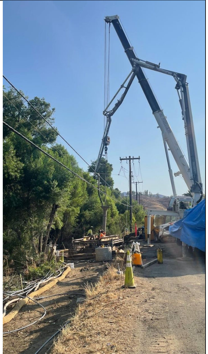
Figure 9. Foundation installation for TSP 370, August 12, 2021
